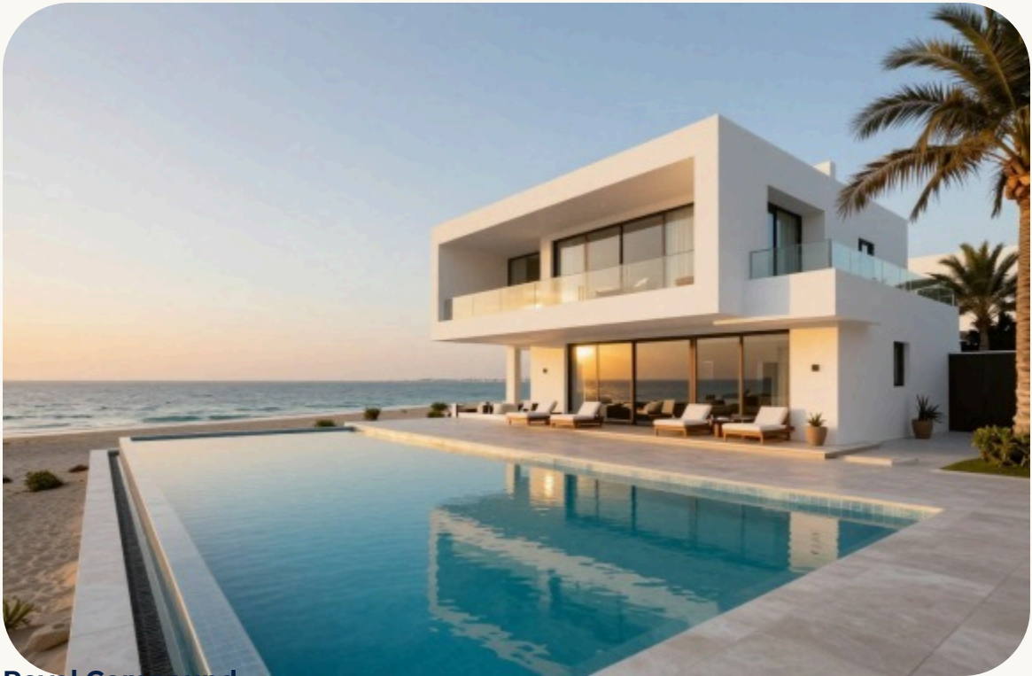
Royal Compound Design-Build | 2,800 sqm
