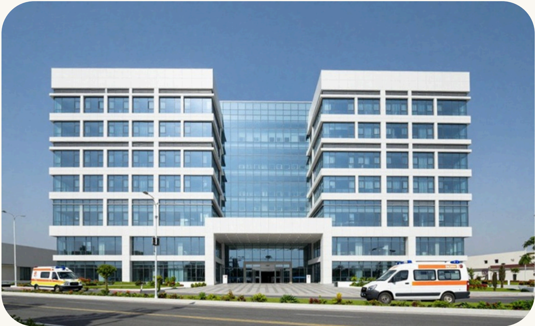
Specialist Medical Centre | Ministry of Health | 8,500 sqm | Full MEP & Finishes
